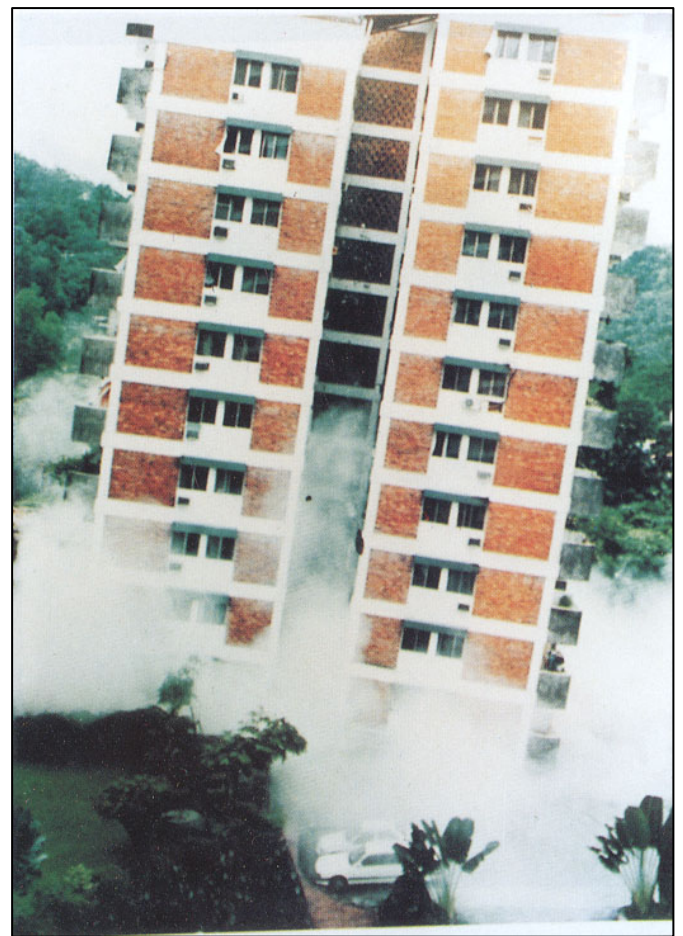
Figure 6 : Block 1 Starts to Topple (from MPAJ, 1994)
