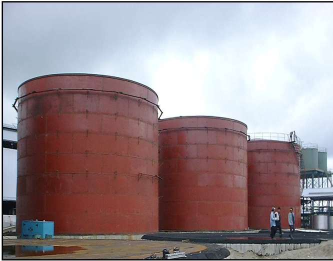
Fig. 46 View of completed tanks.
