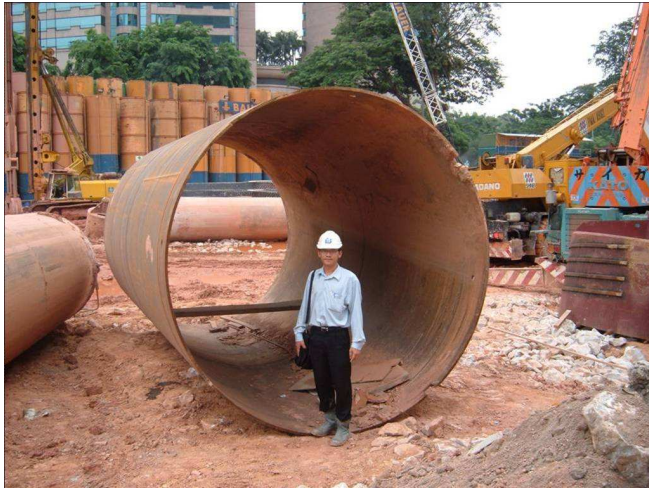
Fig. 3 Casing for 3.0m diameter bored pile.
