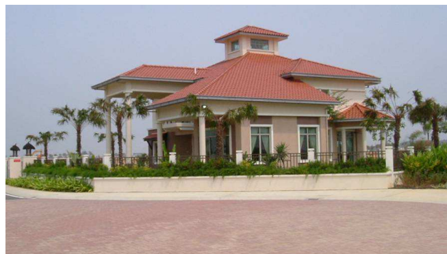
Fig. 40 View of recently completed bungalow houses.
