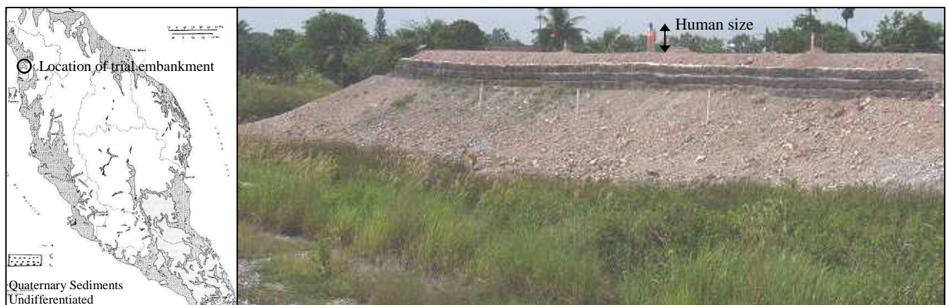
Figure 1 Location and overview of instrumented trial embankment
