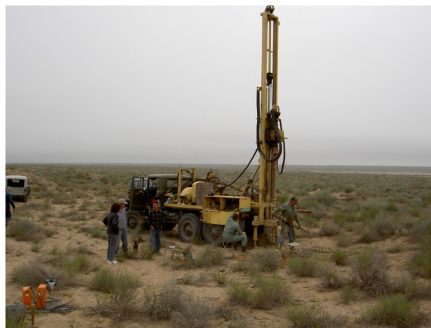
Fig. 25 SI drill rig in Turkmenistan.
