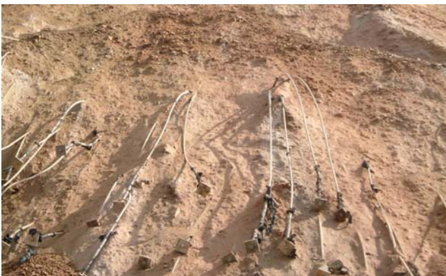
Fig. 11 Example of face failure (front view).
