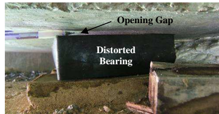
Figure 9 Shearing distortion of rubber bearing
