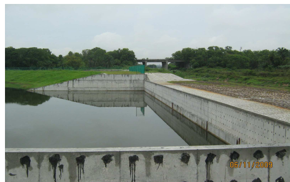
Figure 2 View of the SAS Inlet Structure
