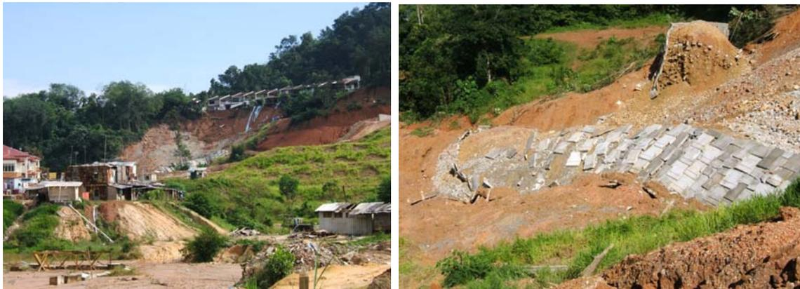
*Collapse of Reinforced Soil Wall at Kampung Pasir on 31 May 2006*
