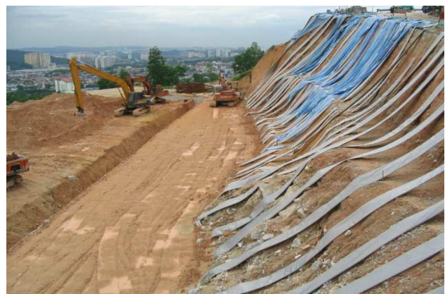
Figure 10 Laying of Strip Drain
