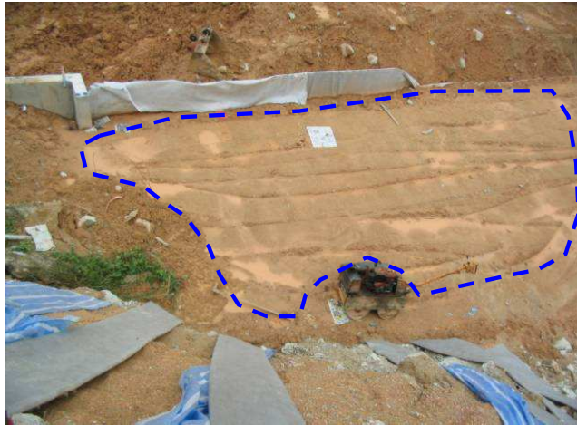
Figure 11 Wet Backfill Material
