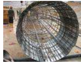
Fig. 7 Double Zinc Sheets wrapped around Test Pile A
