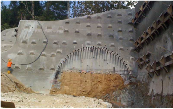
Fig. 4. Soil nailed wall for tunnel face
