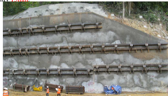
Fig. 3. 15.5m deep excavation with 3 levels of temporary ground anchors
