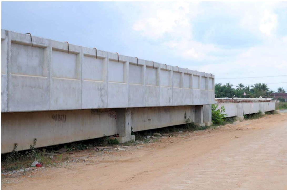
Figure 4: Completed Land Viaduct
